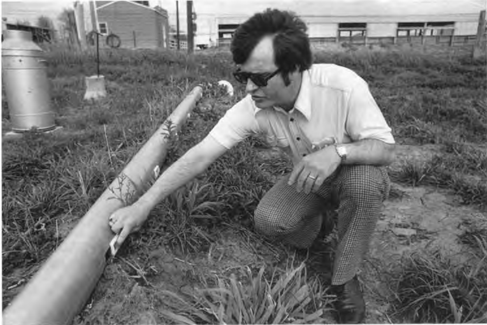
Dale Vanderholm examines the distribution pipe for a feedlot runoff filtration system using vegetative filters.
