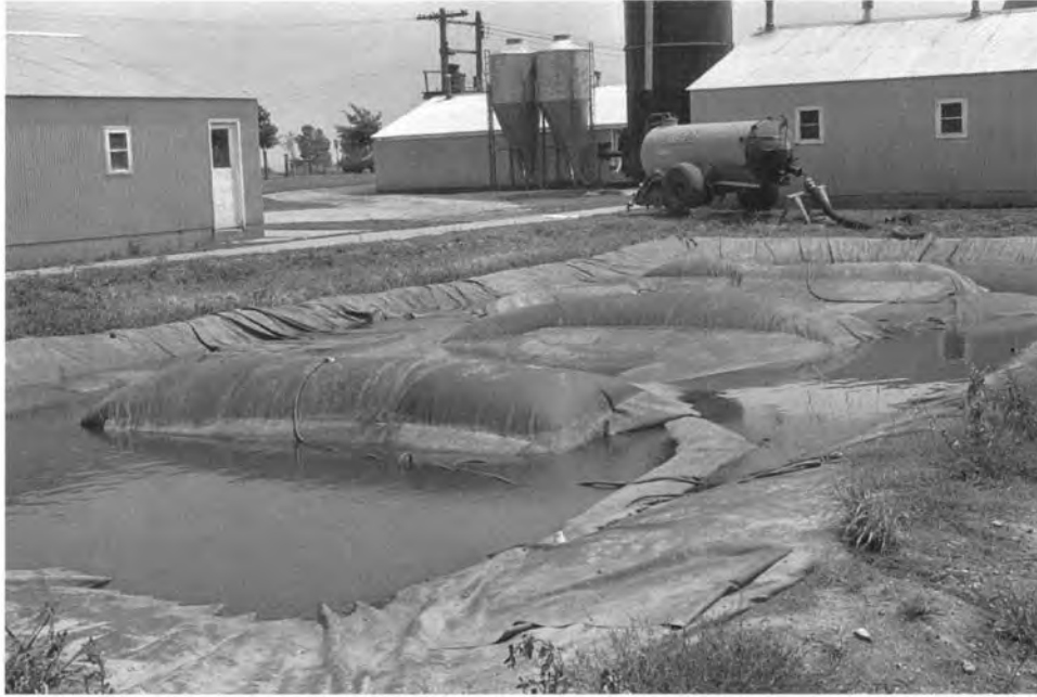
A waste lagoon being developed at the Swine Progeny Testing Laboratory at First Street and St. Mary's Road.
