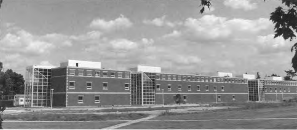
The completed Agricultural Engineering Sciences Building, June 8, 1983.
