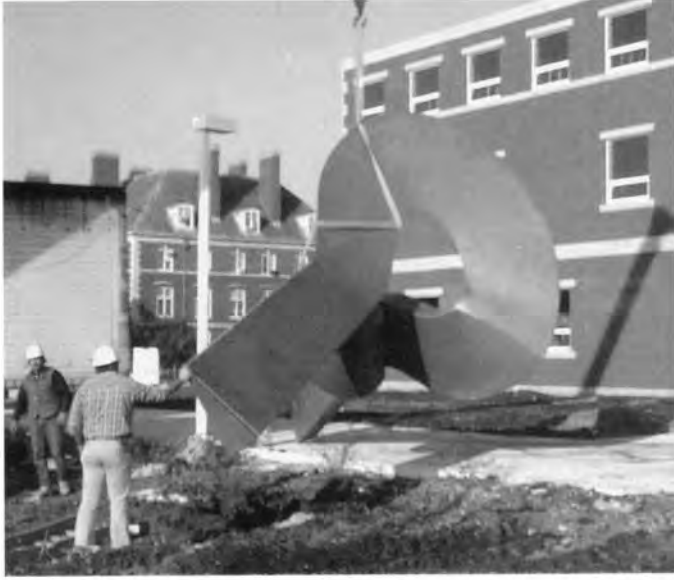
Workmen securing the art piece "Aurora I" by Bruce White into place near the west entrance of the Agricultural Engineering Sciences Building in 1983.
