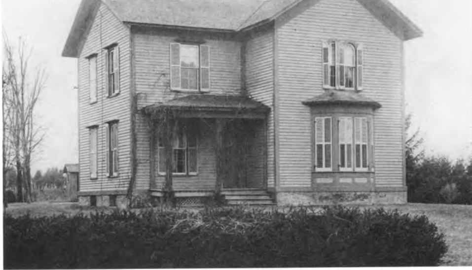
Mumford House, built in 1871, is the oldest building on campus. It was used by Nathan C. Richer in early agricultural mechanization classes as an example of an “improved” farm house. The building is on the National Registry of Historical Places and is currently used by the School of Art and Design.
