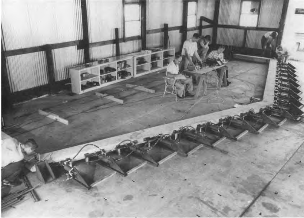
Ed Hansen, Maurice Paul, Charles Spillman, and Jim Curtis, at table, test rigid concrete frames for farm buildings.
